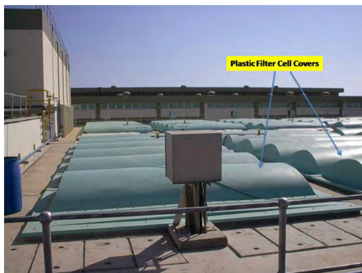
Figure 9.20. Gravity filters protected with plastic covers for control of algal growth showing covers of gravity filters in Ashkelon, Israel.
