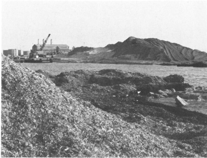
Figure 6.1. Dry seaweed extracted from the Zwitina desalination plant intake channel in Libya. Photo: Kershman 1985.
