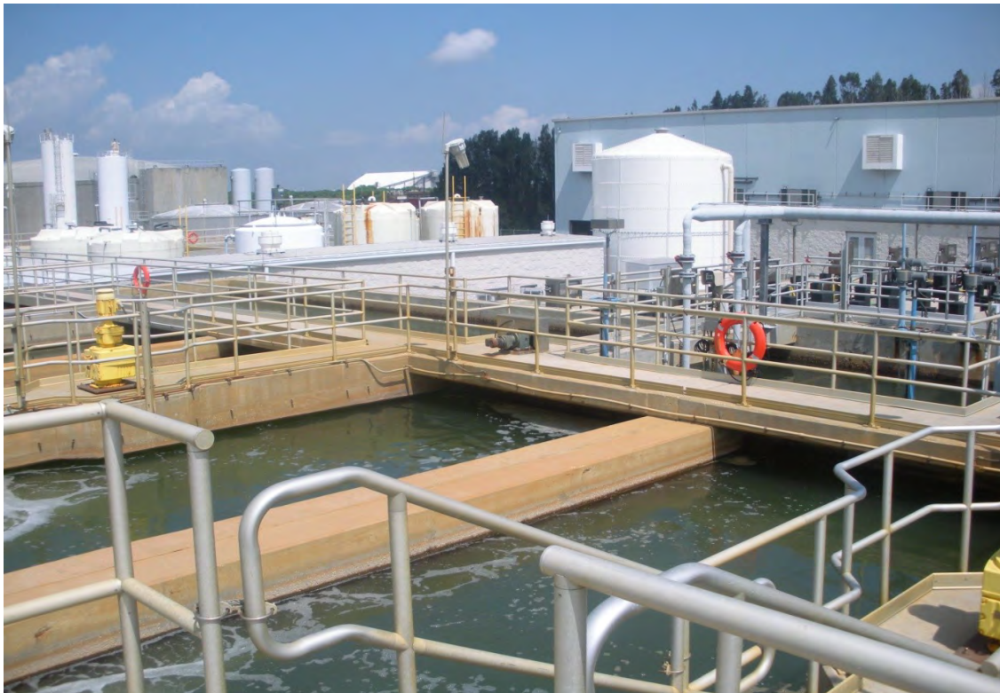
Figure 11.9.3. Normal pretreatment basin appearance (Voutchkov 2009).
