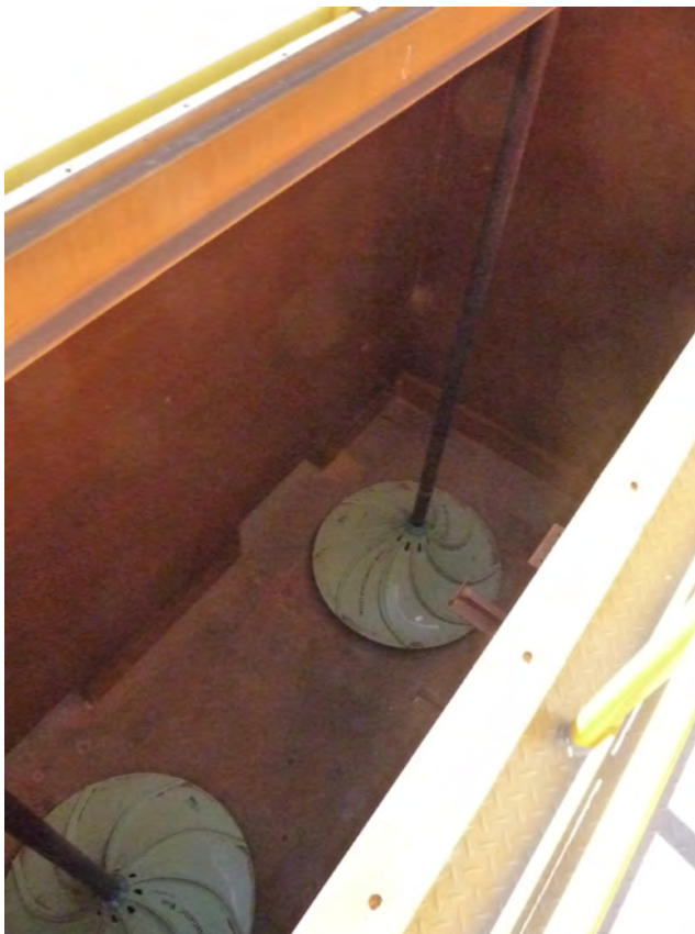
Figure 9.5. Flash mixers in a coagulation tank.
