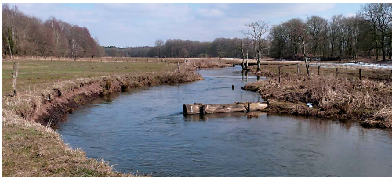
Flow control purposes with coarse woody debris in the river Stör, Schleswig-Holstein
